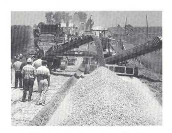
For example, the old slab, rather than being removed and crushed off-site, was required to be crushed and screened in-place, where it would be used as granular subbase. This recycling method was recently developed in lowa by Manatts, Inc. and successfully used for similar work on two Interstate 80 projects east of Des Moines.
