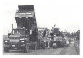
The concrete mix used exhibited good consistency and low slump. Center point beam breaks showed a modulus of rupture well above the minimum 500 psi break specified after 7 days. At 5 specific locations needed to accommodate local services, high-early strength Class "M" concrete that would achieve 500 psi after two days in place was incorporated.
