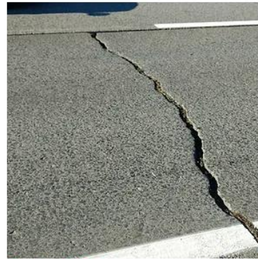
Cracked Slabs
