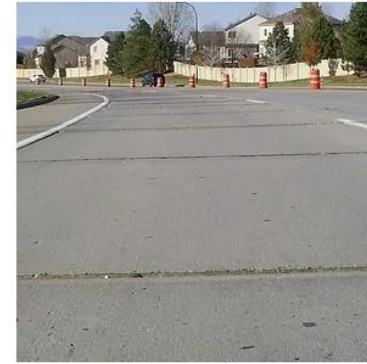
Faulted Joints
